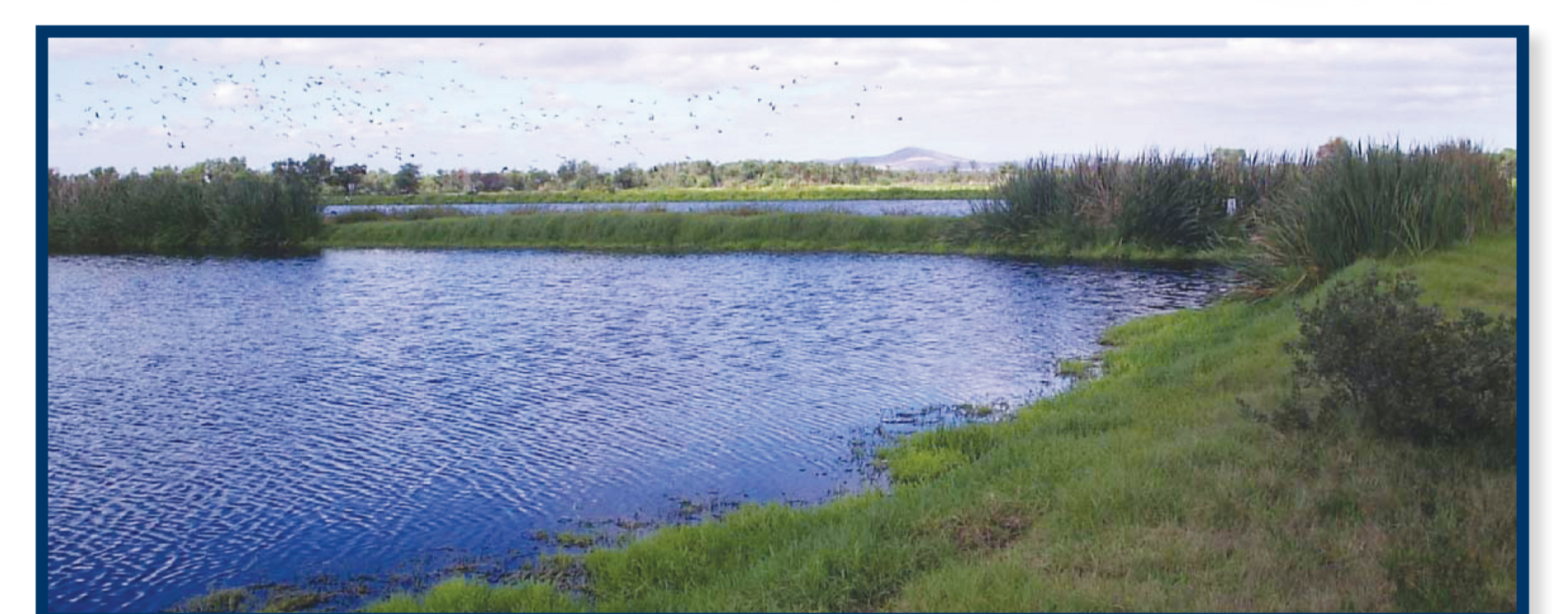
Figure 4: A recharge basin at Atlantis well field, Western Cape, where artificial recharge is being implemented by the City of Cape Town, supported by the CSIR
