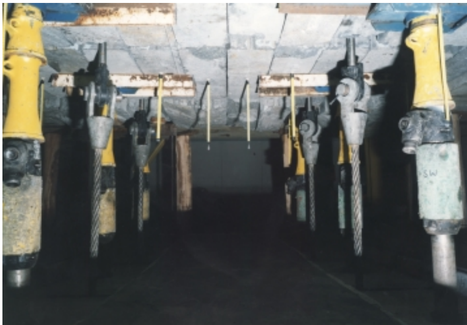
Photograph 5.8 Test # 3, showing asymmetrical location of 800 mm headboards.
