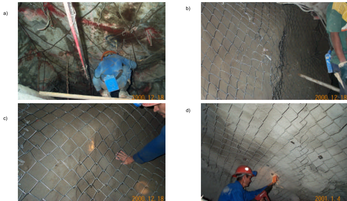
Figure 14: Application of mesh reinforced shotcrete.
