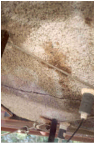
Figure A.49. Shotcrete and lacing 50 cm. drops.
