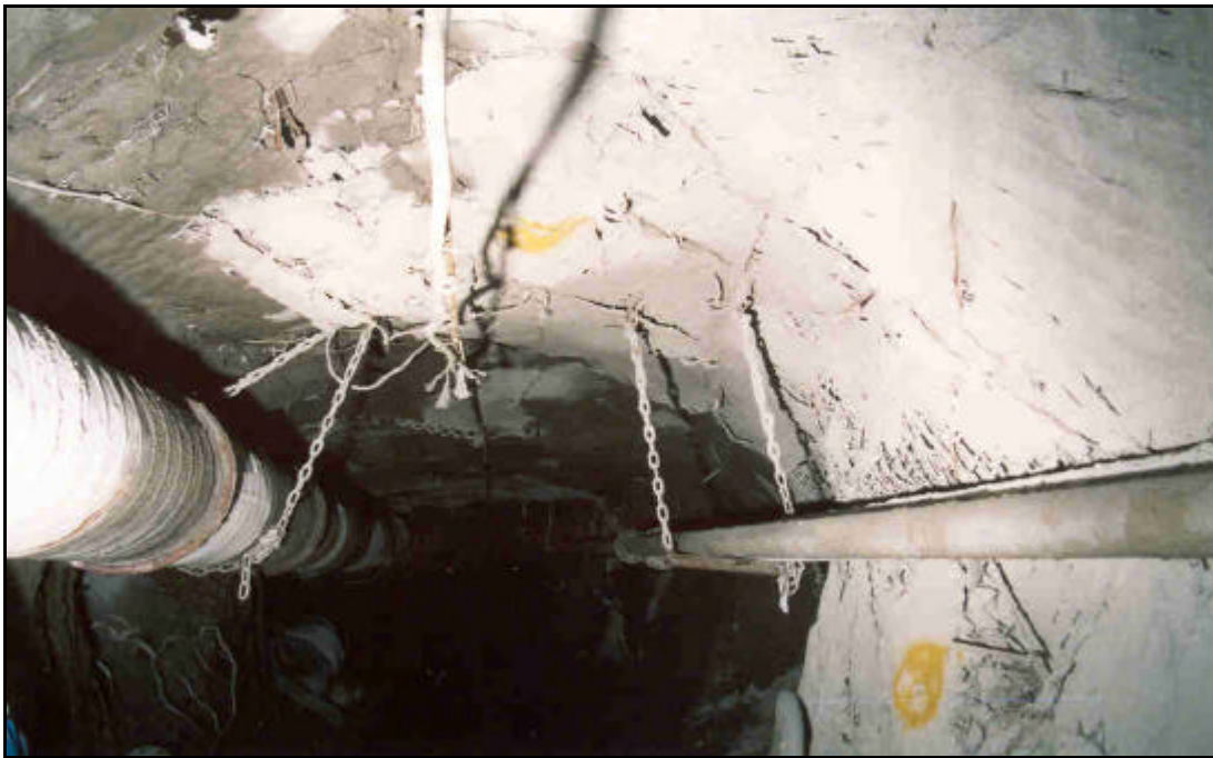
Figure 5.5. Overall tunnel condition around monitoring position 1. (October 2000).
