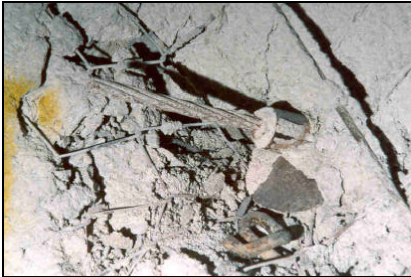
Figure 5.12. Pre-tensioned and post-grouted cable anchor.
