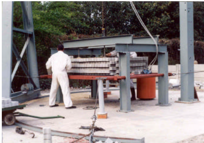
Figure A.2. Preparation of brick assembly.
