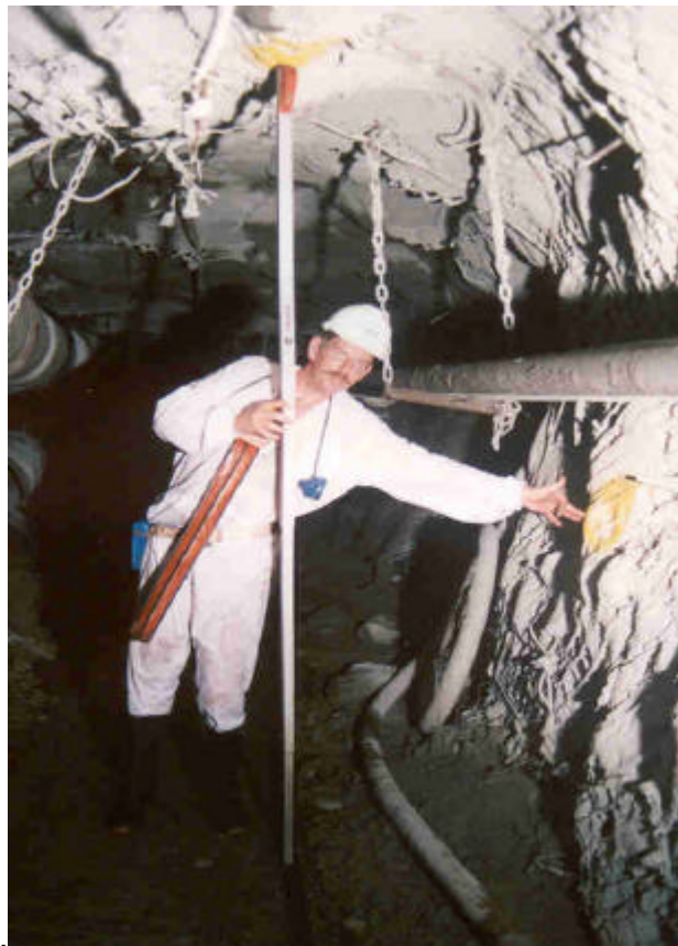
Figure 5.7. Measuring hangingwall – footwall closure at monitoring position 2.
