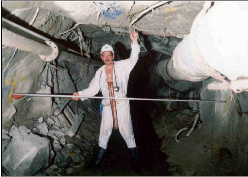
Figure 5.6. Overall tunnel condition around the monitoring position 2.
