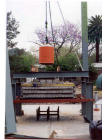
Figure A.3. Brick assembly completed.
