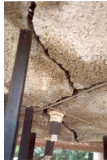
Figure A.48. Shotcrete and lacing 50 cm. drops.
