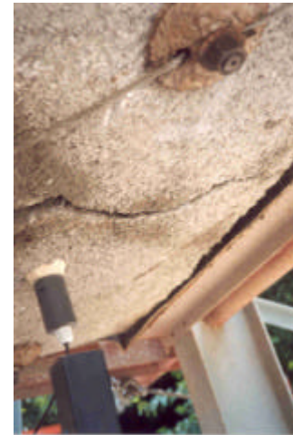
Figure A.51. Shotcrete and lacing 50 cm. drops.
