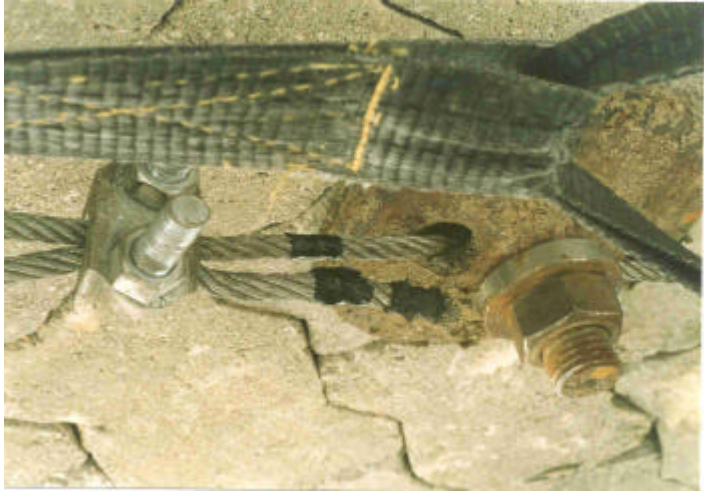
Figure A.41. Detail of lacing.
