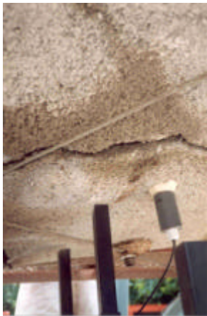
Figure A.50. Shotcrete and lacing 50 cm. drops.
