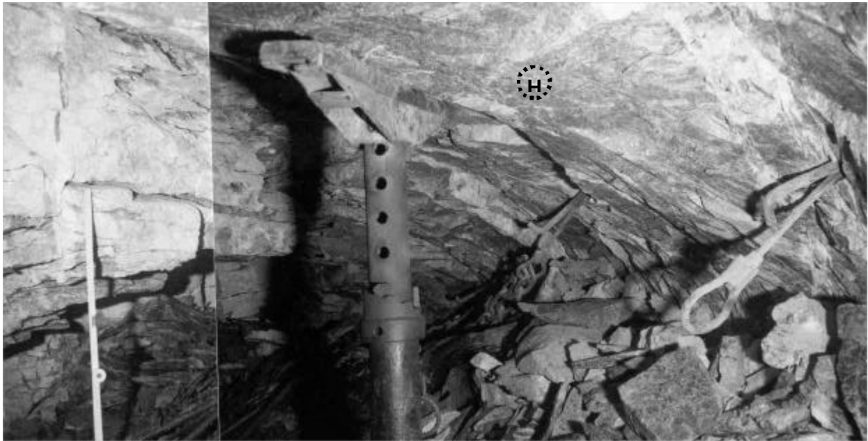
Figure 4.2.6 Hangingwall-parallel fractures (H) arching down to siding face in 102 stope at Tau Tona mine
