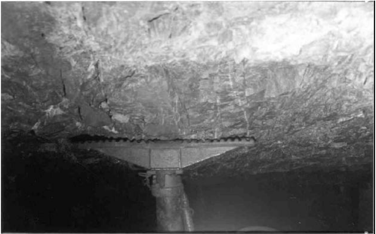
Figure 4.2.7 Steep dipping, stope-face parallel fractures in second panel away from pillar in 102 stope at Tau Tona mine
