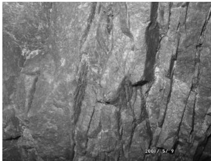
Figure 4.5.6 Photograph of steeply dipping fractures in hangingwall of 'window 1', (5 m from face) 50-25 E5 gully at Driefontein 5 Shaft
