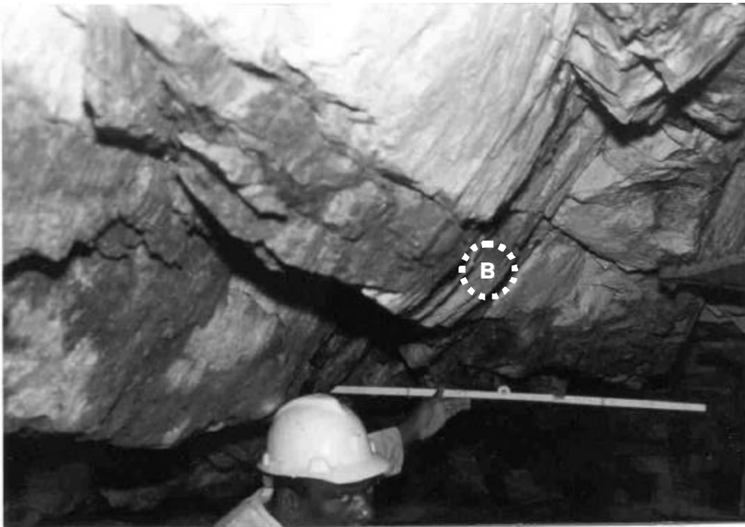
Figure 4.4.2 Hangingwall at bottom of E1 panel, 94-48 VCR stope at Mponeng mine: exhibiting dominant backward-dipping fracturing (B) (face at right)
