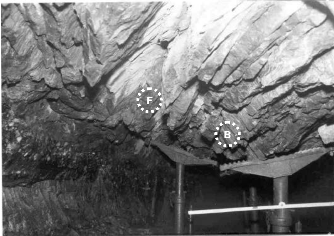
Figure 4.4.3 Hangingwall up dip from the bottom of E1 panel, 94-48 VCR stope at Mponeng mine: exhibiting dominant forward-dipping fracturing (F) and minor backward-dipping fracturing (B) (face at left)
