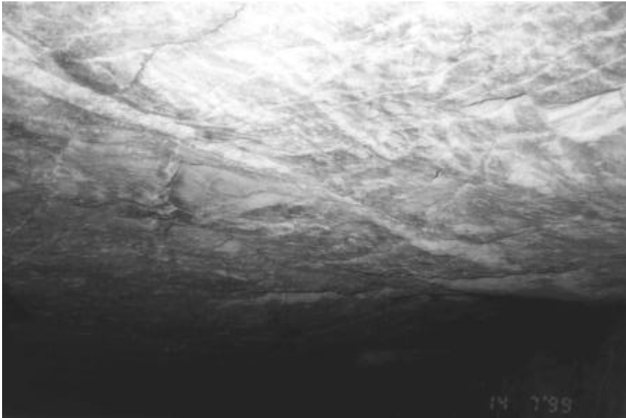
Figure 4.1.2 Smooth hangingwall conditions in a backfilled stope at Kopanang mine
