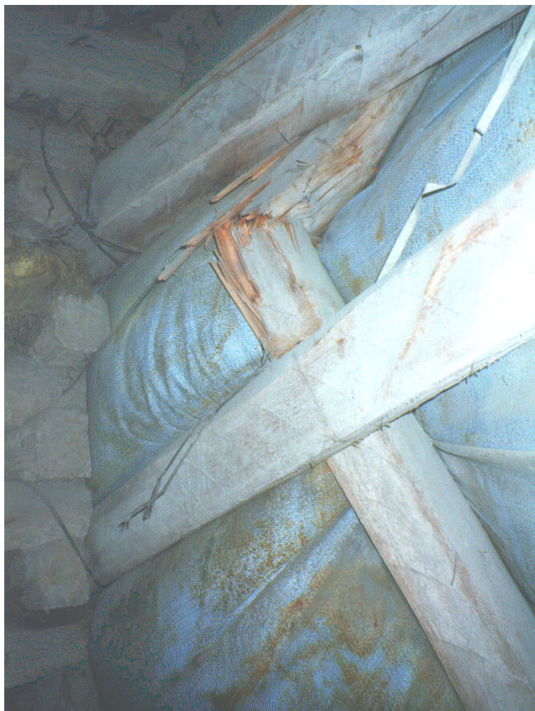
Figure 2.7 Closure on backfill in the back area.
