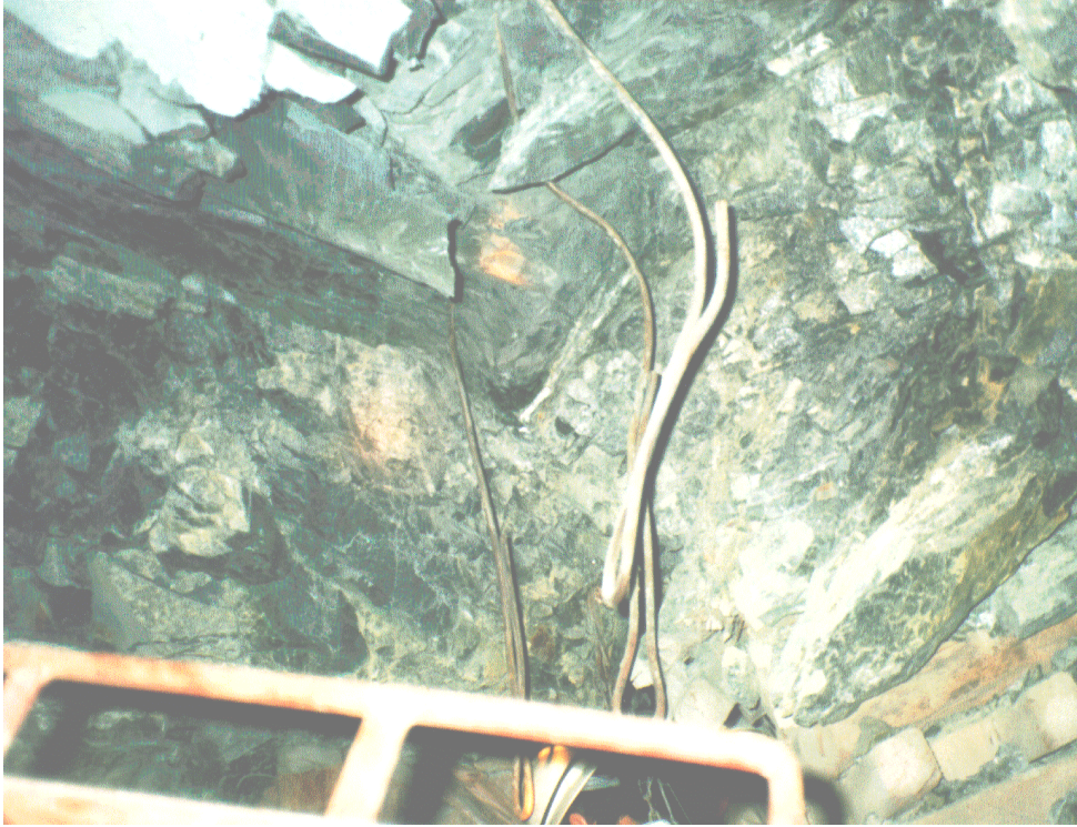
Figure 2.3 Buckling of the Greenbar in the gully hangingwall.
