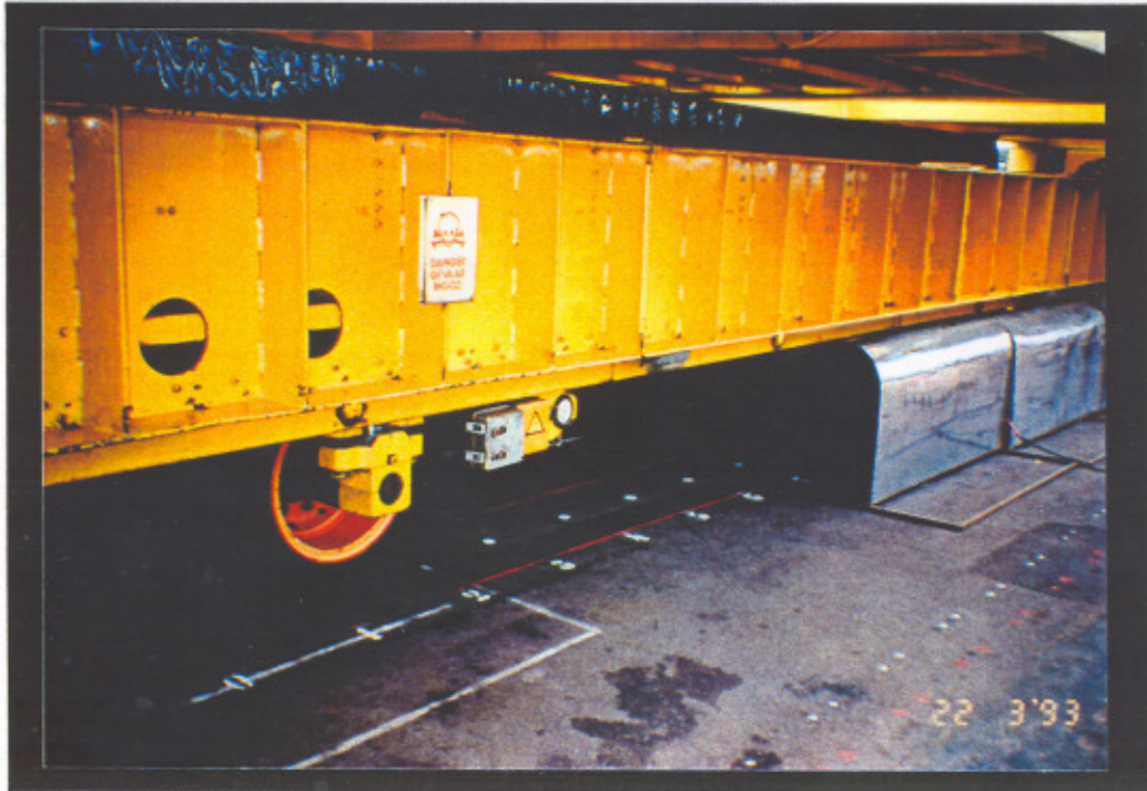
PHOTOGRAPH 4 : Heaters used to elevate the temperature in the asphalt mix
