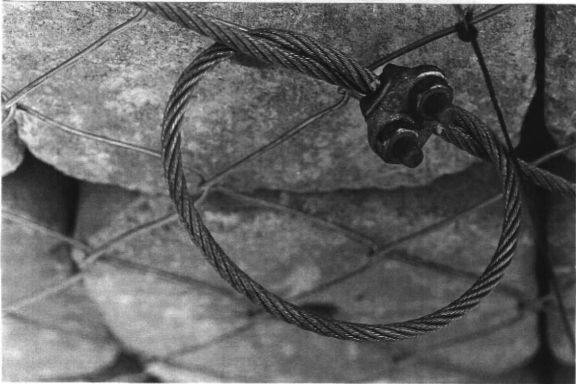
Photo 12: Test No. 43. Impulse of 37,3 kJ caused complete collapse. Detail of northern loop before impact. One Crosby clamp at low torque.
