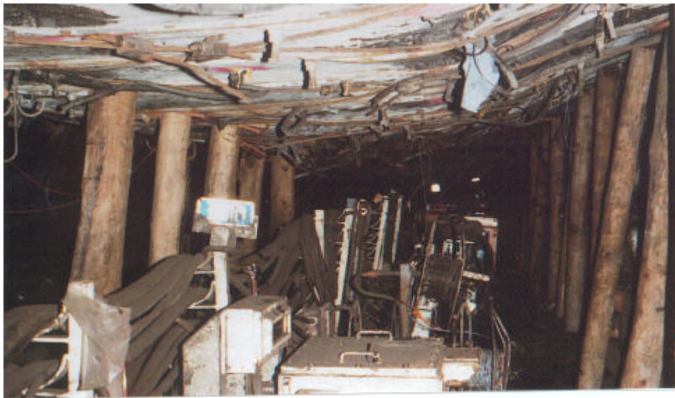
FIGURE 5.1 Mining Conditions Associated with Adverse Horizontal Stress Effects (Australia)
