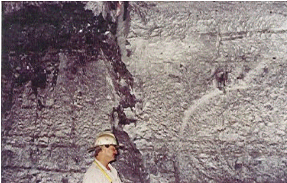
FIGURE 4.10. Open Jointing Observed During Mine Site Inspection
