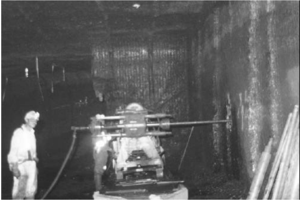
Figure 4–3 Photograph of site with drill rig in place at pillar 3.
