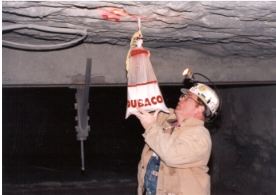
Figure 5.1c: Installation of individual stone dust bag in crosscut
