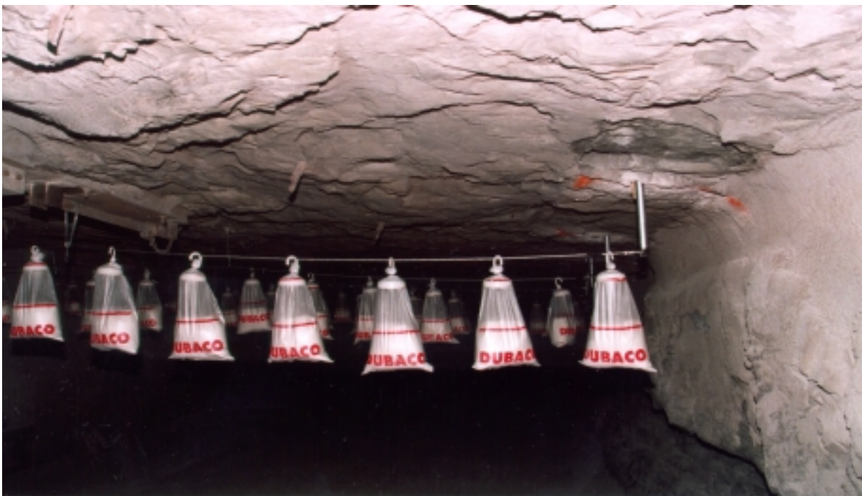
Figure 5.2.3b: Stone dust bags suspension method
