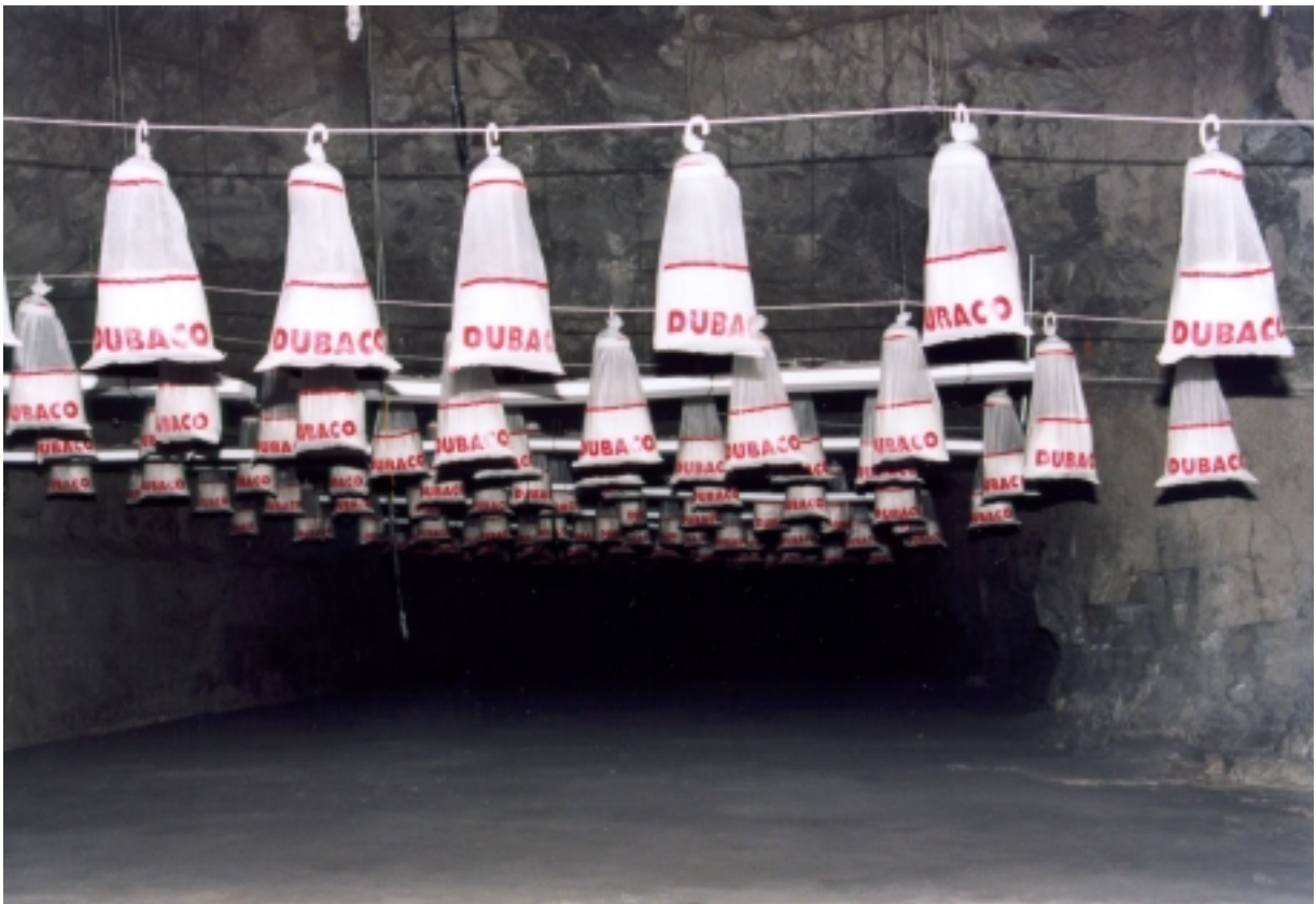
Figure 5.2.5a: Concentrated barrier installation in B-drift
