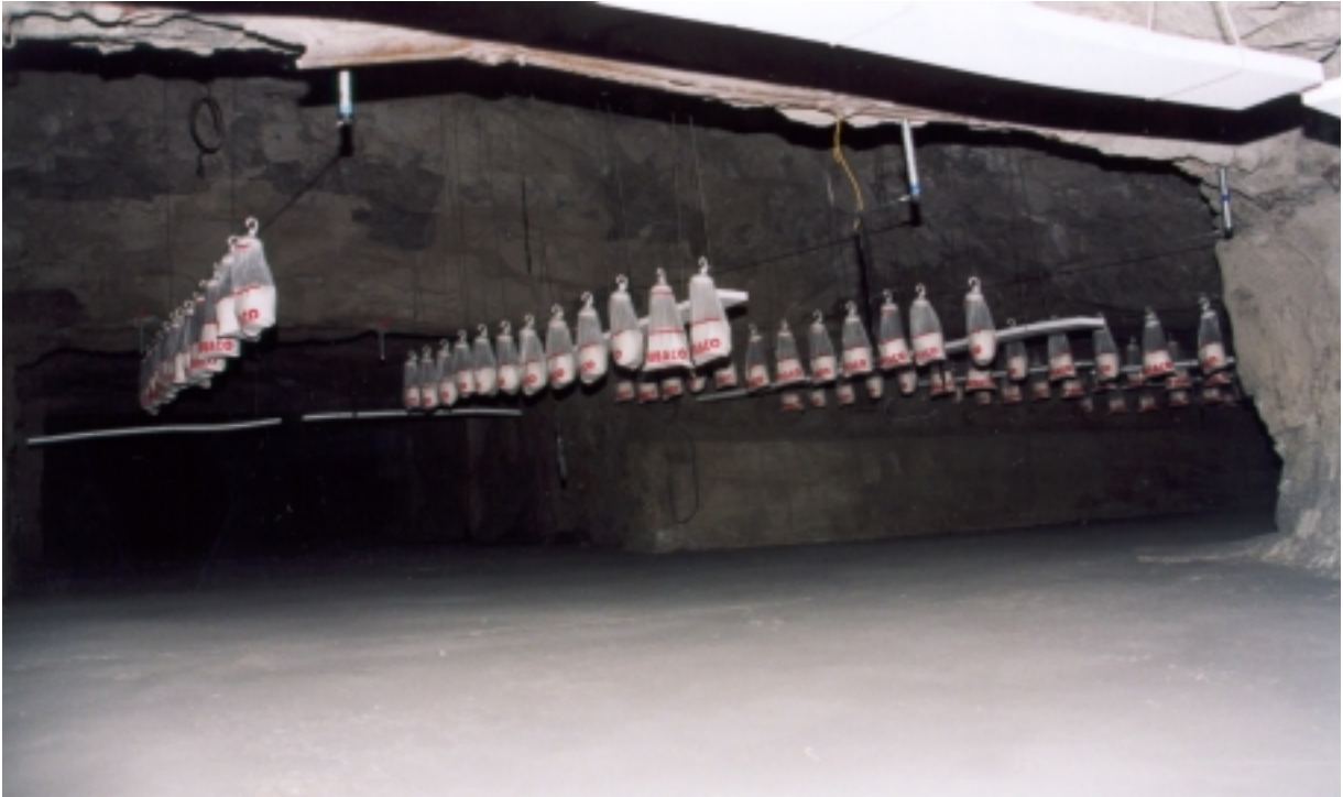
Figure 5.2.5b: Concentrated barrier installation in B-drift, as viewed from the crosscut
