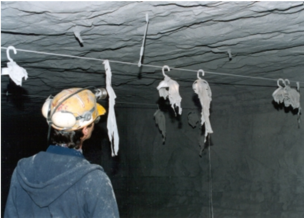
Figure 8.2.2c: Photograph of remnants of bags at the fourth sub-barrier
