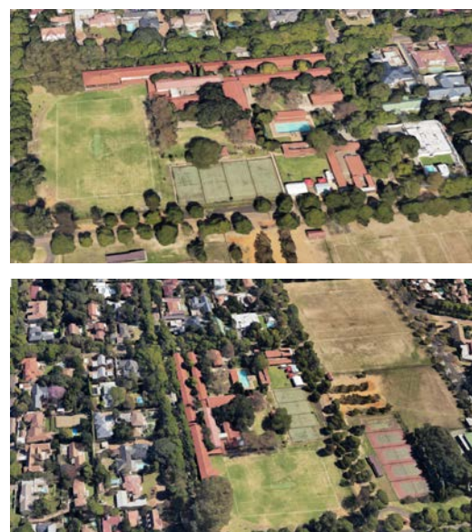
Figure 5. Photographs of Case Study School in Pretoria, Gauteng
