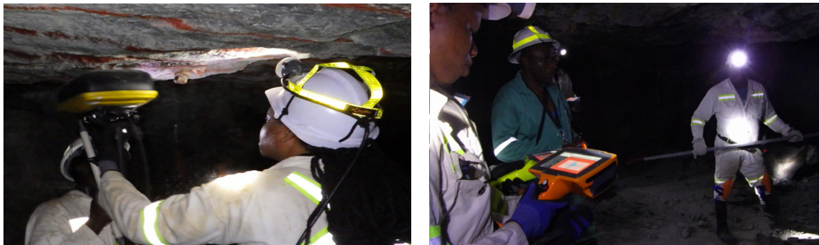
Figure 2. Trials of (a) Ground penetrating radar (GPR), (b) Integrated thermal and acoustic device (ITAD).
