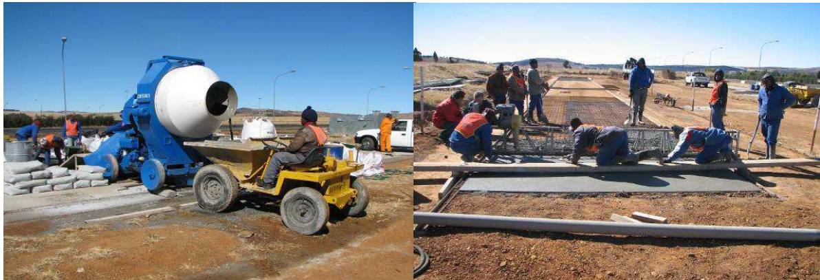
Figure 17: Mixing and Placement of Phase 2 UTCRCP
