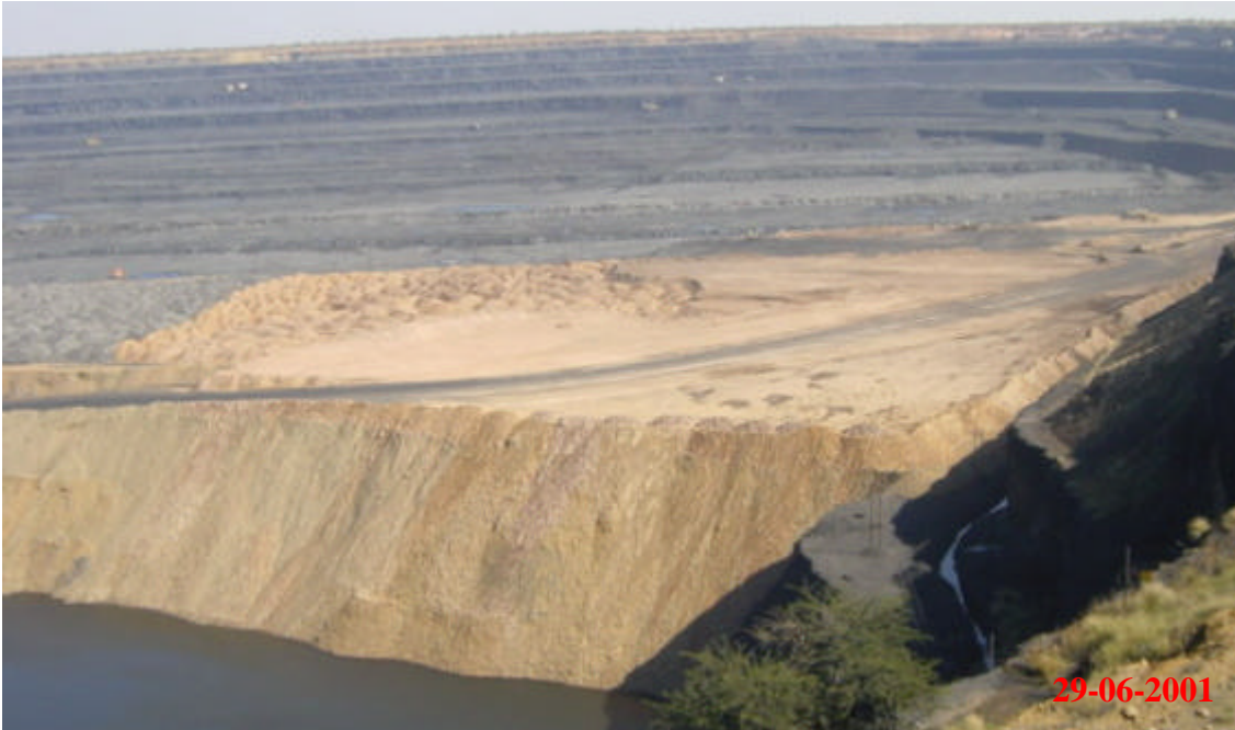
Figure 5.8: First-year Compartment, Surface-sealing of Sub-level 1C
