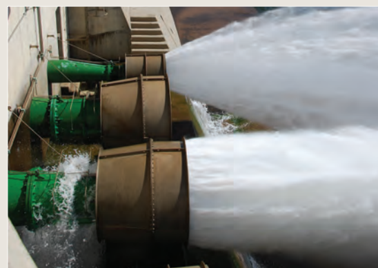
Reserve (small outlet ) and irrigation (larger outlet) water being released downstream during April 2011.
