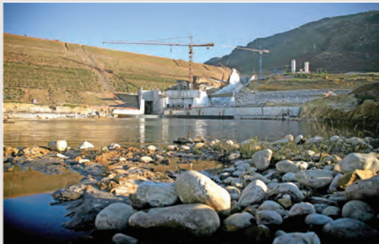
The Berg River Dam under construction with (l. to r.) the rectangular flood release conduit, duplicated small and larger outlets at centre for Reserve and other low-flow releases, and the spillway
