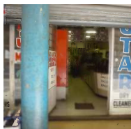
This picture shows a large threshold from the street into the shop. The shop itself has a highly reflective slippery tile floor.
