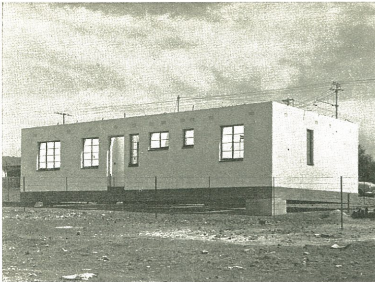
Above: Experimental house built on three concrete pads — one at each back corner and one in front centre; it is hoped that this construction may overcome effects of expanding (heaving) clay foundations which cause severe wall cracks in many areas.
