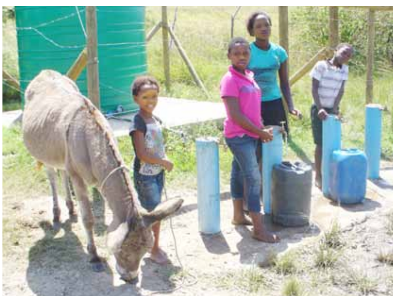
Children from the nearby community collecting safe, sustainable drinking water from taps. The water is pumped from the communal water station to a small storage tank, from where gravity carries the water in pipes all the way to taps in the village.
