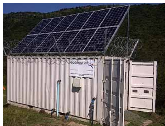
Various renewable and alternative energy supply options were investigated for the communal water stations. Solar power, as seen at this communal water station, with diesel generators as back-up was found to be the most suitable.
