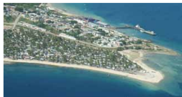
Pictured is the highly vulnerable area at the north-western tip of the city of Pemba in Mozambique, where the village of Paquite is regularly threatened by sea inundation.
