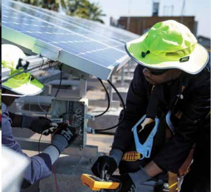
Above and left: CSIR intern Siyasanga May inspecting the wiring of the photovoltaic testing facility at the CSIR. The CSIR is developing wiring standards for photovoltaic facilities.
