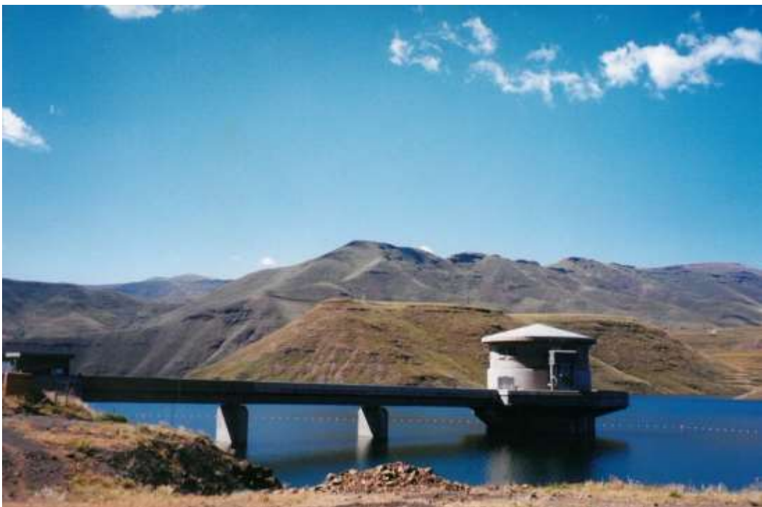
Figure 5: Outlet from the Katse Reservoir (Photo courtesy of Suzan Oelofse)
