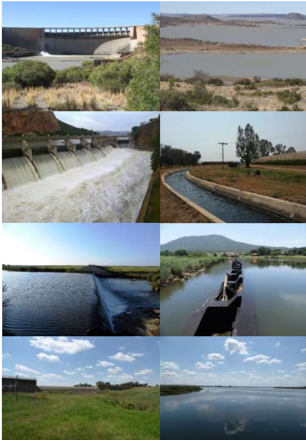
Figure 1: Some of the large water infrastructure successive South African governments and private entities have constructed to cope with times of drought. The Gariep Dam and its extensive reservoir (top) on the Orange River supplies much needed water to the Eastern Cape to sustain the Province's agricultural, domestic and industrial economic sectors through an inter-basin transfer scheme (photos courtesy of Wilmot Webster). The Hartbeespoort Dam supplies water to the Hartbeespoort Irrigation Scheme (second from the top) and Hartbeespoort and Brits towns. A weir on the Olifants River (middle left) supplies water to
