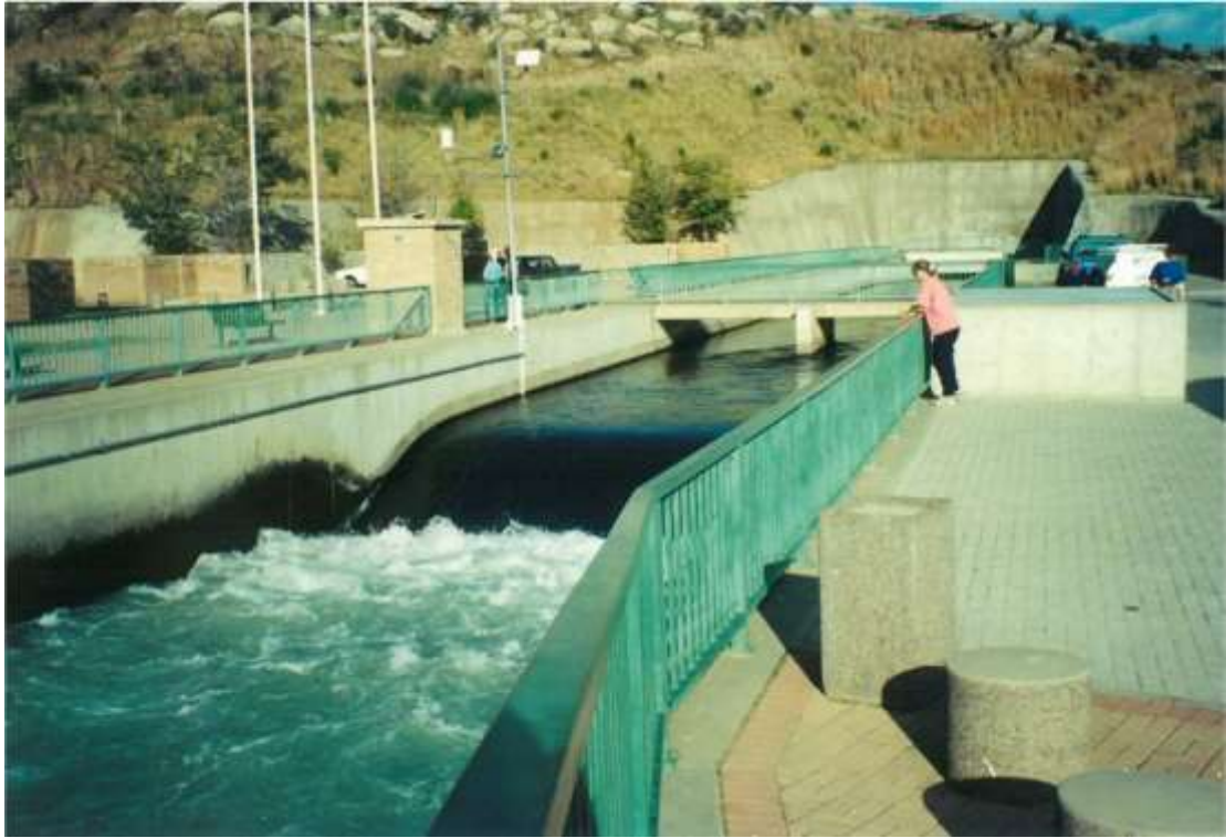
Figure 6: Water from the Katse Reservoir in Lesotho arriving at the outfall to the Ash River in the eastern Free State, South Africa (Photo courtesy of Suzan Oelofse)
