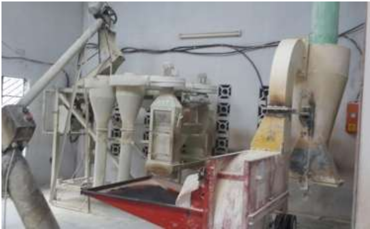
Figure 214: The mill where the maize bran comes out from the mill
