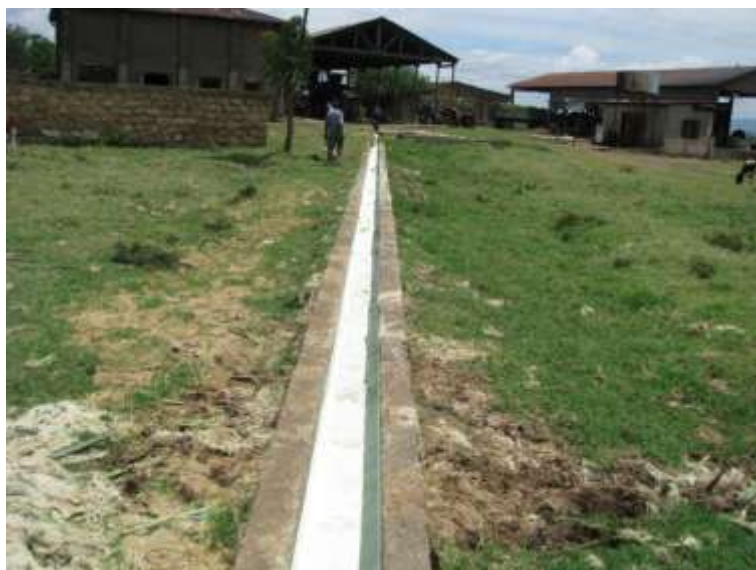
Figure 143: Athinai Sisal factory. The channel is where the watery residue from pressing the sisal is transported for disposal.
