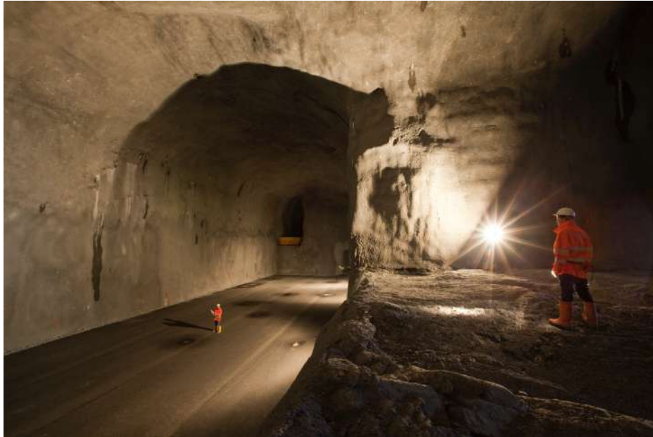
Figure 5: Human made cavern in Switzerland designed for industrial production. Source: Amberg Engineering AG.
