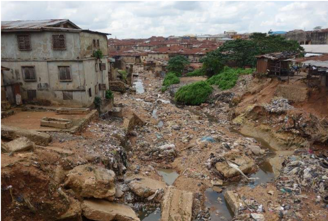
Figure 2.2 The build-up of waste in the river system is an issue in Ibadan
