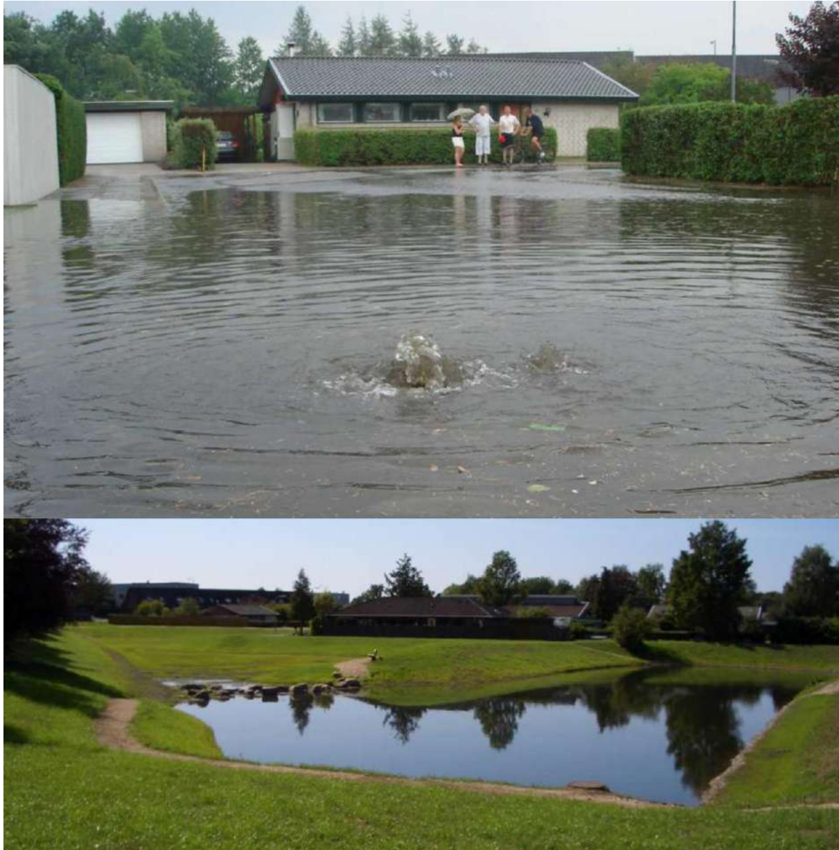
Figure 4: From problem to solution. Above: re-occurring flooding in residential areas in Odense city. Here from Ejersminde Street. The citizens themselves came with the proposition to turn the most challenged areas into a storm water basin that also functions as a recreational area for the neighbourhood (Laursen & Linderberg, 2017). Photo: Ejgil Juul Nielsen.
