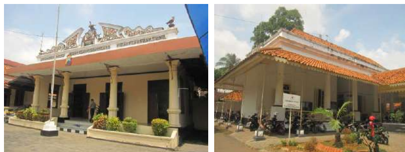
Figure 4. Building of Dutch epoch was function-transfered into Administrative Office (Source: Private Document, 2018)
