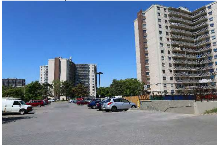
Figure 1: A view of the apartment towers on one of the candidate sites (Site A)
