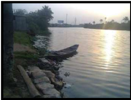
Photo 1: Inadequate setback of houses
