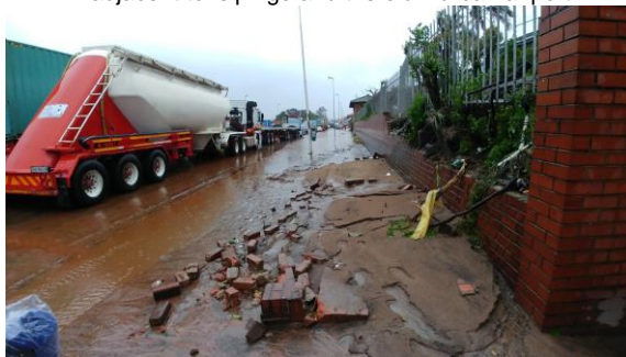
Collapsed wall outside King Edward Hospital in eThekweni 16
