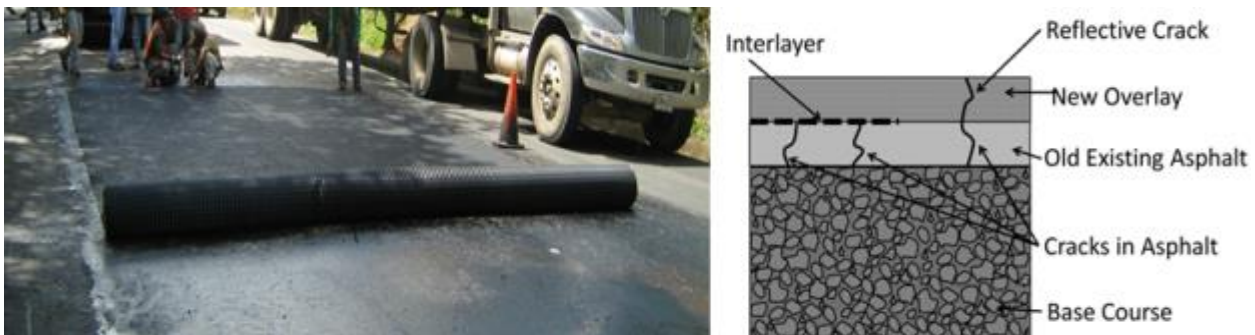
FIGURE 2 Geogrid Interlayer Reinforcement and HMA Overlay Construction.
