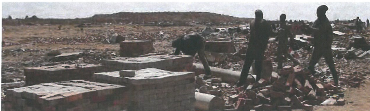
Reclaiming bricks from a landfill in the City of Tshwane, South Africa
