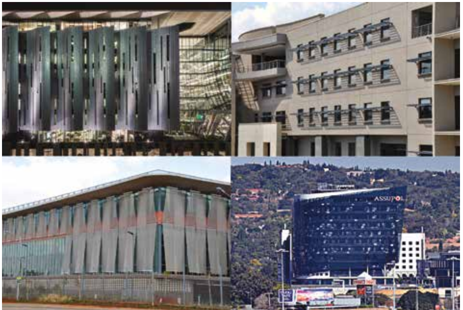
Figure 7: Examples of solar protection in South Africa. The building top left used vertical fins to protect a north-eastern facade. The building top right used small horizontal solar protection inappropriately on the western façade. Bottom left and right illustrate two types of solar shielding screens on the building northern facades.
