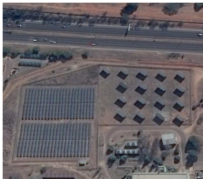
Figure 3: Google Earth image of the single axis tracker and the adjacent 202 kWp DC dual-axis plants at the CSIR Pretoria campus.
