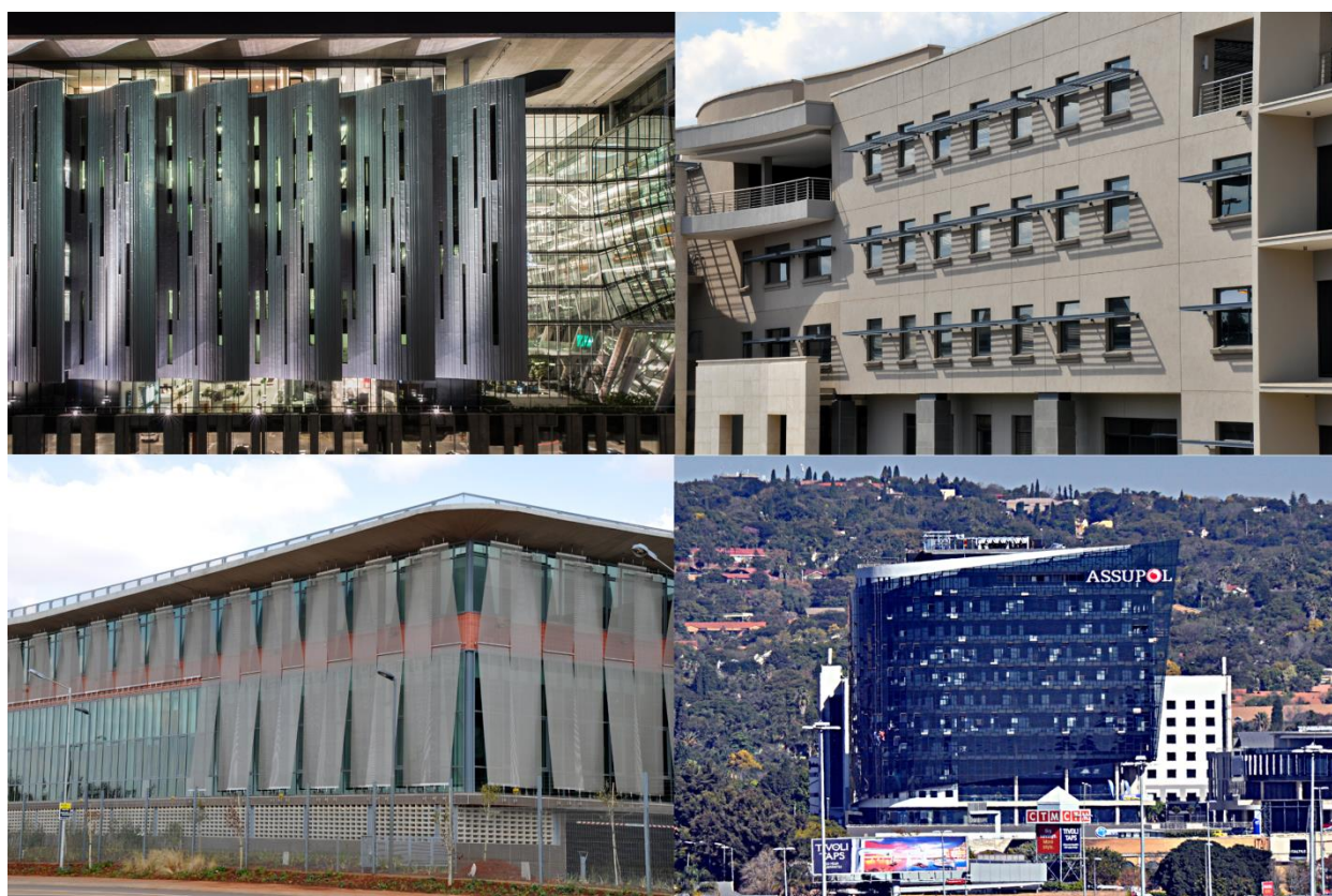
Figure 7: Examples of solar protection in South Africa. The building top left used vertical fins to protect a north-eastern facade. The building top right used small horizontal solar protection inappropriately on the western façade. Bottom left and right illustrate two types of solar shielding screens on the building northern facades.
